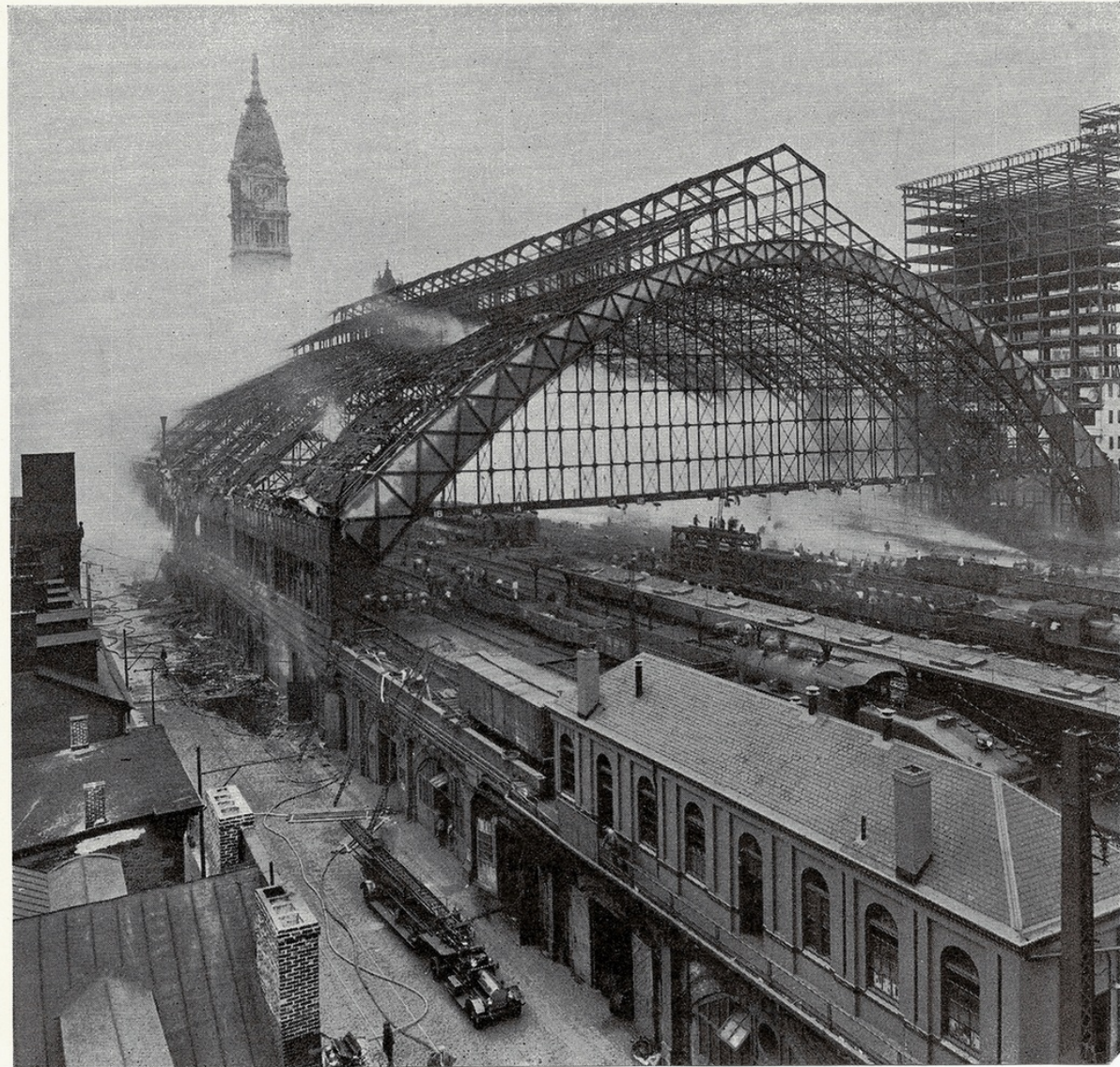
The remains of the train shed with City Hall in the background; the ladder fire engine is on Filbert Street. Work crews are starting reconstruction even as the station smoulders. The building under construction on the right is the Fox Theatre.
