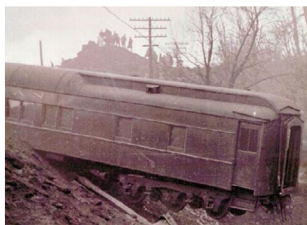
A passenger car hanging over the rim of the curve. Greg Sheets - Altoona Archive
