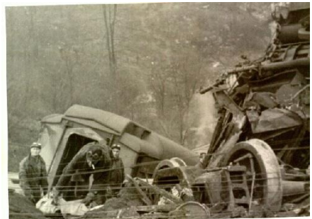
Closeup of workers among the wreckage. Greg Sheets - Altoona Archive
