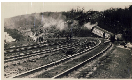
Looking into the curve with wreckage on the right. www.tunnelhillboro.com
