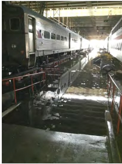
MEADOWS MAINTENANCE COMPLEX CAR SHOP
