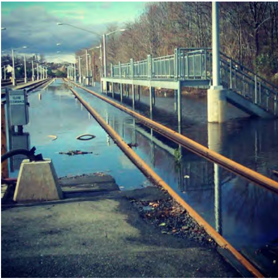
NEW JERSEY TRANSIT BAY HEAD, NJ PIT TRACK
