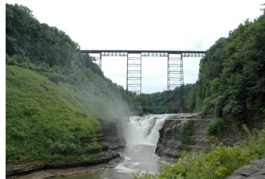
PORTAGE BRIDGE AS IT APPEARS TODAY
