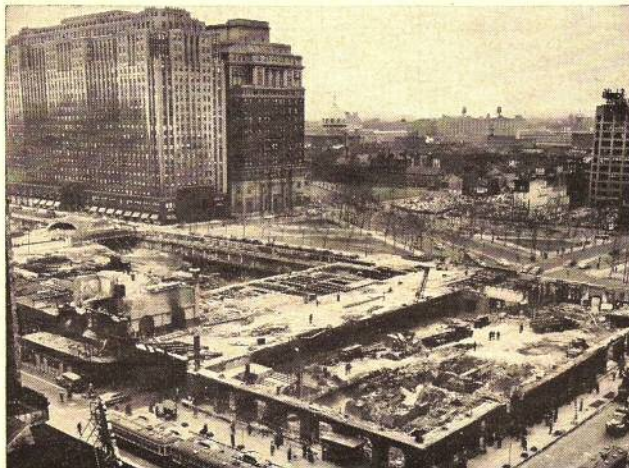
Eleven months later: Only the concourse floor, part of southwest tower, and the walls of Old Broad's ground floor remain
