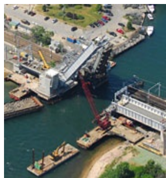
NEW NIANCTIC RIVER BRIDGE WITH 1907-BUILT BRIDGE ADJACENT.
