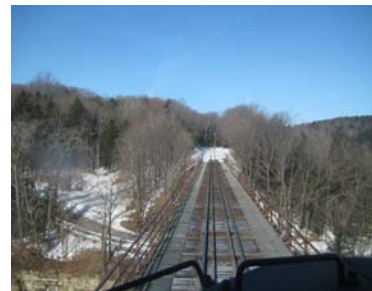
LOCOMOTIVE ENGINEER'S VIEW OF THE PRESENT PORTAGEVILLE BRIDGE
