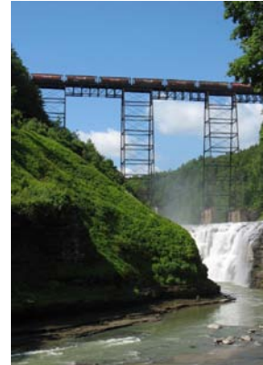
PRESENT PORTAGEVILLE BRIDGE
