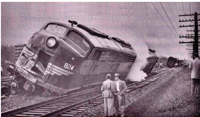
REMNANTS OF THE HORRIFIC TRAIN/TANK ACCIDENT ON THE ERIE TRACKS NEAR FAIRVIEW AVENUE. IT'S THOUGHT THAT THE GENTLEMAN WEARING THE FEDORA IS JAMES W. CONNOR, KENT DIVISION TRAINMASTER. ERIE NO. 824 WOULD BE REBUILT AND SERVE INTO THE CONRAIL YEARS AS NO. 4013. (AKRON BEACON JOURNAL FILE PHOTO)
