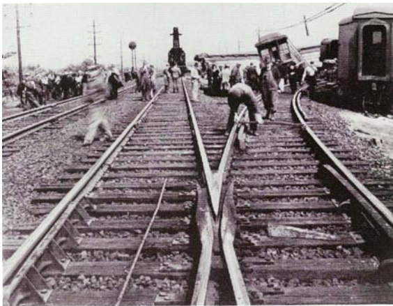
Train No. 1080 derailed upon entering the sharp curve of the Minson connecting track at Delair. The scene of the wreck taken the following morning shows switch No. 25 in the foreground. Note the man checking the gauge of the connecting track.
