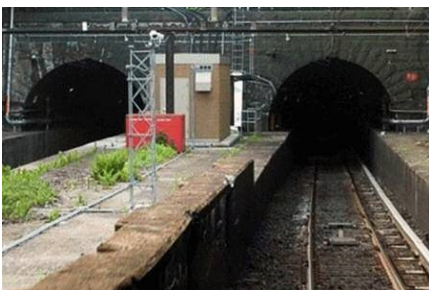
THE EXISTING HUDSON RIVER TUNNELS ARE MORE THAN 100 YEARS OLD AND REQUIRE SERVICE OUTAGES EVERY WEEKEND TO PERFORM ROUTINE MAINTENANCE - AMTRAK
