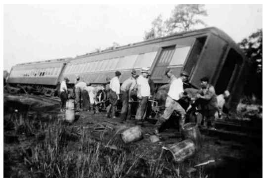
A CREW FROM THE CENTRAL RAILROAD OF NEW JERSEY WORKS TO UPRIGHT THE DERAILED BLUE COMET THE DAY AFTER THE WRECK ON AUG. 19, 1939. HERBERT AND EDITH GERBER COURTESY OF ROBERT GERBER JR.
