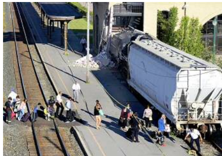
AMTRAK PASSENGERS ARE ESCORTED AROUND THE DAMAGED UTICA UNION STATION ON JULY 21, 2015 TINA RUSSELL, UTICA OBSERVER-DISPATCH
