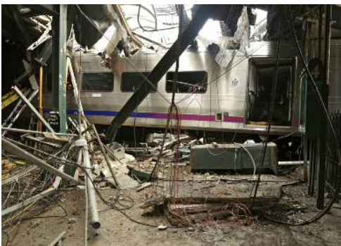
NJ TRANSIT WRECKAGE IN THE HOBOKEN TERMINAL SHOWN IN AN IMAGE FROM THE NATIONAL TRANSPORTATION SAFETY BOARD
