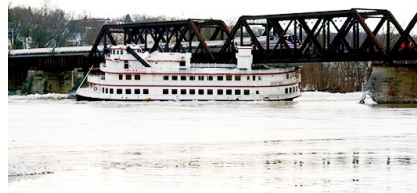
AMTRAK EMPIRE SERVICE TRAIN 281 FROM NEW YORK PENN STATION TO NIAGARA FALLS, N.Y., CROSSES THE LIVINGSTON AVENUE BRIDGE IN ALBANY, N.Y., AS THE CAPTAIN JP III CRUISE SHIP REMAINS WEDGED AGAINST THE BRIDGE ON FRIDAY, JAN. 25 - DAN KITTAY
