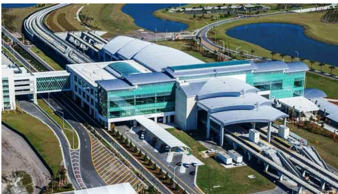
A RENDERING OF THE VIRGIN TRAINS STATION AT ORLANDO INTERNATIONAL AIRPORT PHOTO – VIRGIN TRAINS USA
