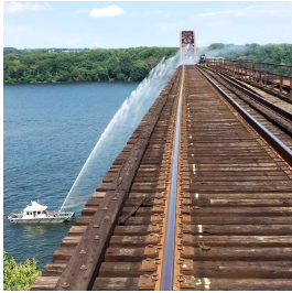
CREWS FROM THE SUSQUEHANNA HOSE COMPANY ARE SHOWN FIGHTING A FIRE ON THE CSX RAILROAD TRACKS CROSSING THE SUSQUEHANNA RIVER BETWEEN HAVRE DE GRACE AND PERRYVILLE. (COURTESY SUSQUEHANNA HOSE Co.)
