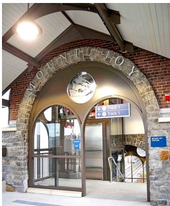
GUESTS ARE GREETED BY THIS ARCHED GATEWAY UPON ARRIVING AT THE NEW MOUNT JOY STATION - DAN CUPPER
