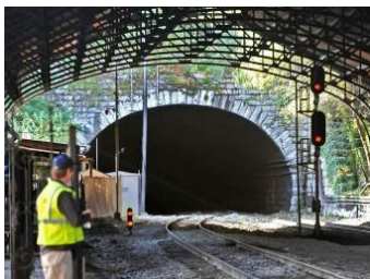
CSX HOWARD STREET TUNNEL
