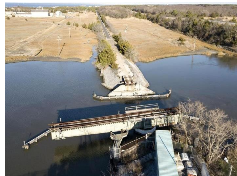
THE RAILROAD SWING BRIDGE IN THE LEWES-REHOBOTH CANAL WITH THE FORMER RAIL BED HEADING TOWARD THE DELAWARE BAY. PHOTO BY NICK ROTH, CAPE GAZETTE
