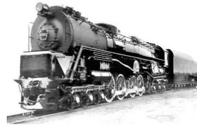
**Mar. 26, 1945** - Class S2 6-8-6 steam turbine locomotive placed in revenue service between Chicago and Crestline; normally running east on *The Trail Blazer* and west on *The Admiral*.
