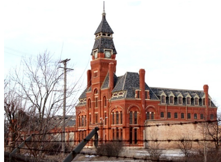
THIS BUILDING WILL BE THE HOME OF THE PULLMAN NATIONAL MONUMENT VISITORS CENTER, EXPECTED TO OPEN IN 2021 - BOB JOHNSTON
