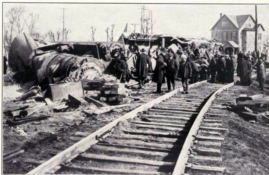
FIG. 1.—General view of scene of accident. Derailed engine, lying on its side, and forward cars of the train. Track with tie rods; tie-plated, and double-spiked, inside
