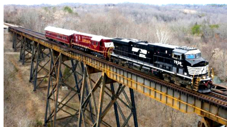
NS AUTONOMOUS TRACK INSPECTION IS NOW MOUNTED ON THE LOCOMOTIVE. PHOTO VIA NS.
