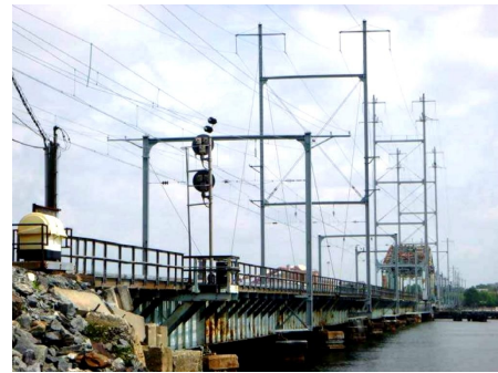
EXISTING RARITAN RIVER BRIDGE
