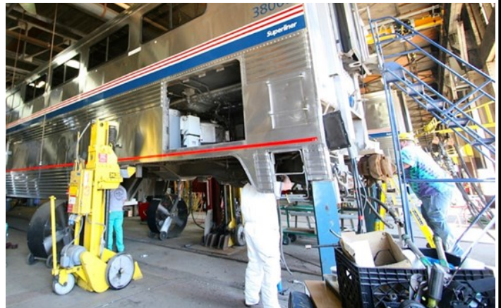
Amtrak workers at Beach Grove Indianapolis rebuild a Superliner dining car in 2026.
