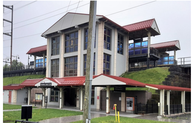
Pennsauken Transit Center
