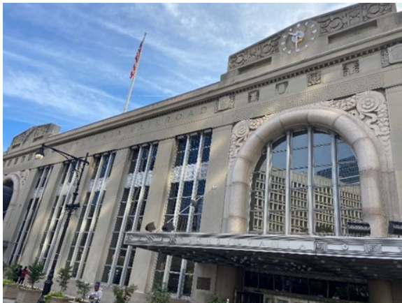
Newark NJ Penn Station Front Facade
