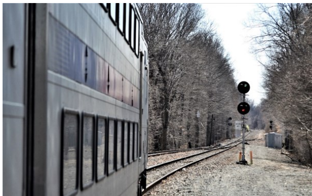
Left: Signal at High Bridge, looking East – photo by Bruce Adams
