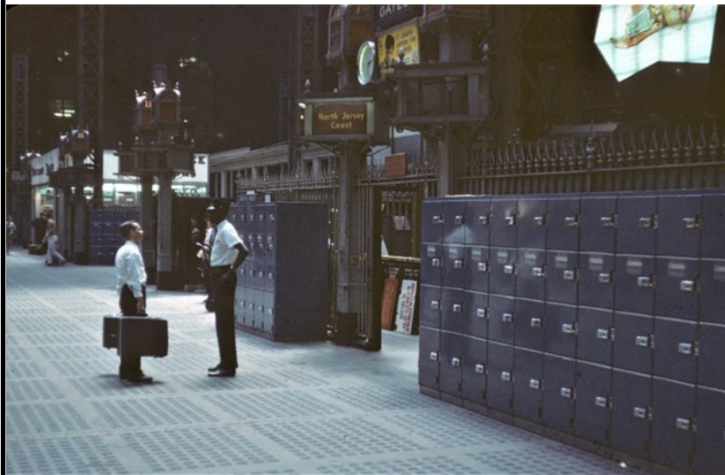
Photo of the passenger concourse and gates of the original Penn Station from the early 1960's. Used with permission of the Railroad Museum of Pennsylvania. (from the Ira Silverman slide collection)
