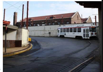
Overhead trolley and bus turnaround loop
