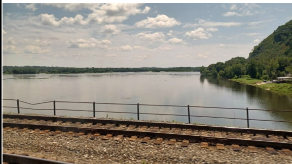
Above, the Susquehanna River from the famed Rockville Bridge
