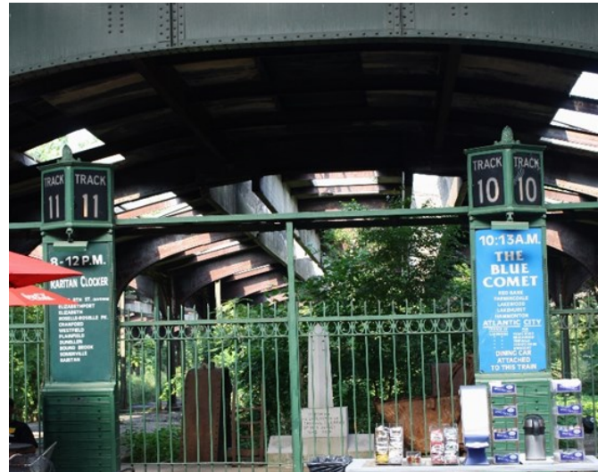
Former boarding concourse of the Blue Comet in a recent photograph. The gates and the bush shed over the former tracks still exists, however the tracks have all been removed – Photo by author
