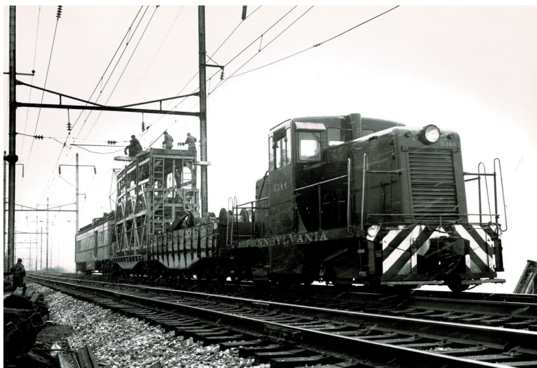
The Lancaster Wire Train at Washington Boro on the A&S Branch on December 26, 1956. PRR 9344 GE 44T is the motive power.
