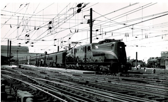
PRR GG1 at Washington Union Station ca. 1935 H.W. Pontin photo
